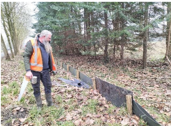
Leen v. Brakel repareert paddenscherm © C.Vermeulen
